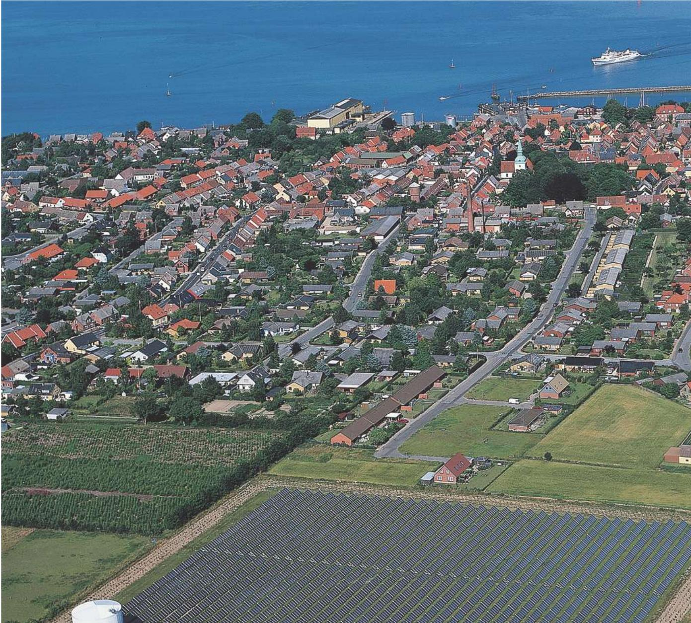
18,000 m<sup>2</sup> collectors help to heat the small town of Marstal, popn. 3,000. Large solar collector fields produce heat at one-fifth the cost of heat from collectors on house roofs.
