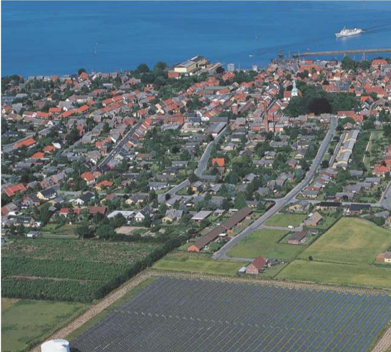
1996/2002 – 18,000 m<sup>2</sup> of ground-mounted solar collectors and a seasonal heat store help to heat the small coastal town of Marstal. Heat network temperatures were dropped to 70/40°C to raise the solar fraction.
