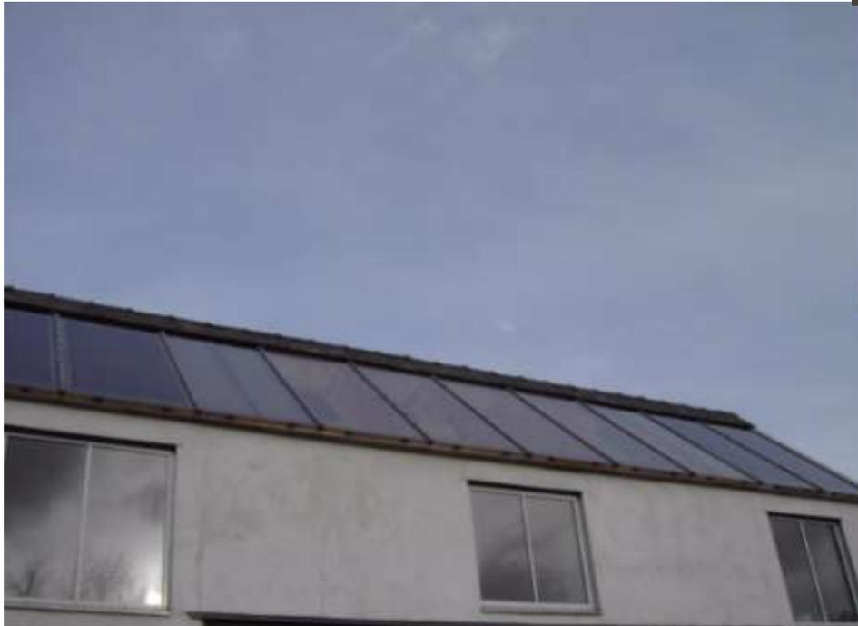
The project will eventually produce all its energy from solar, mainly passive gains, an experimental solar water heating system and roof-integrated photovoltaics.
