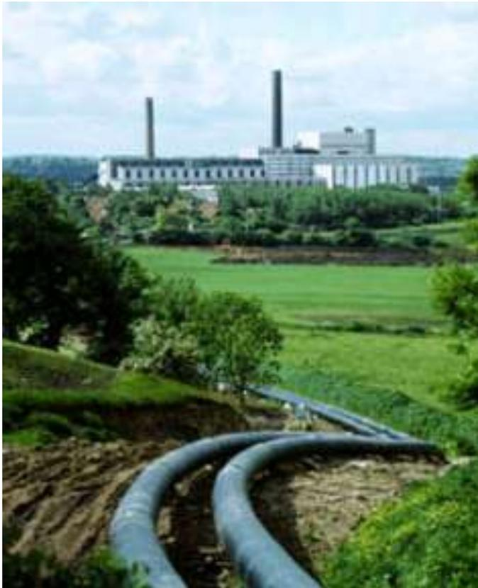
*Top right* - cross-linked polyethylene twin pipe developed for use in low-density areas; e.g., suburbia.
