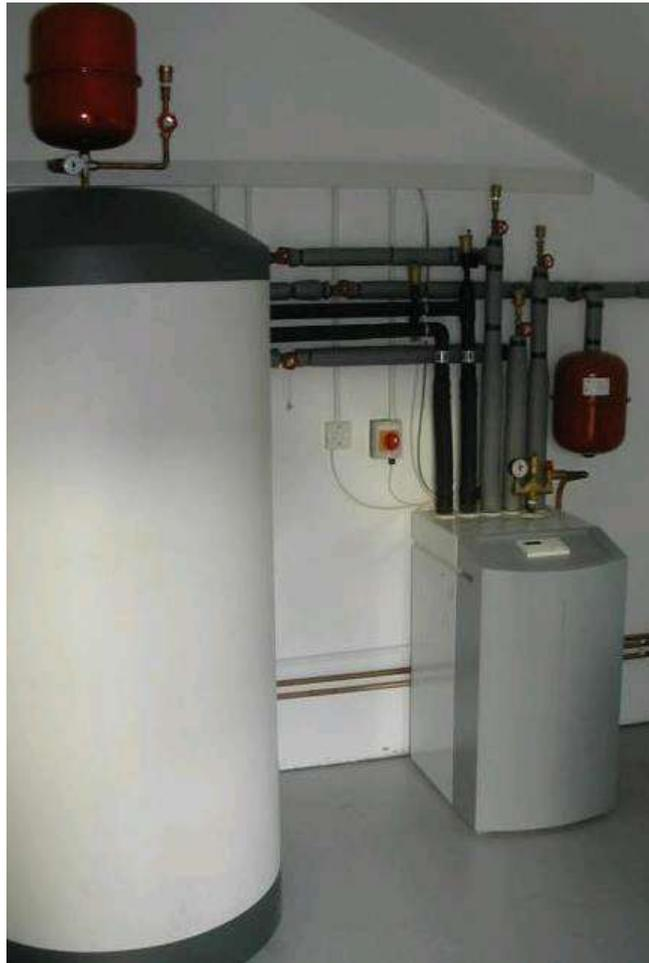
*Below left and top right - 10 kW(t) spring source system, Wales with a 700 litre buffer store.*
