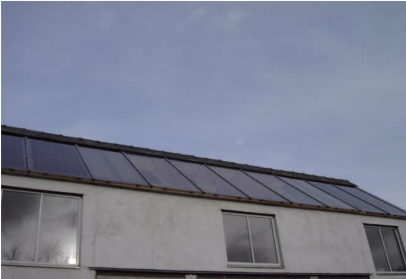
The glazing bars between the panes are stainless steel. This has a lower embodied energy than the more common aluminium bars.
