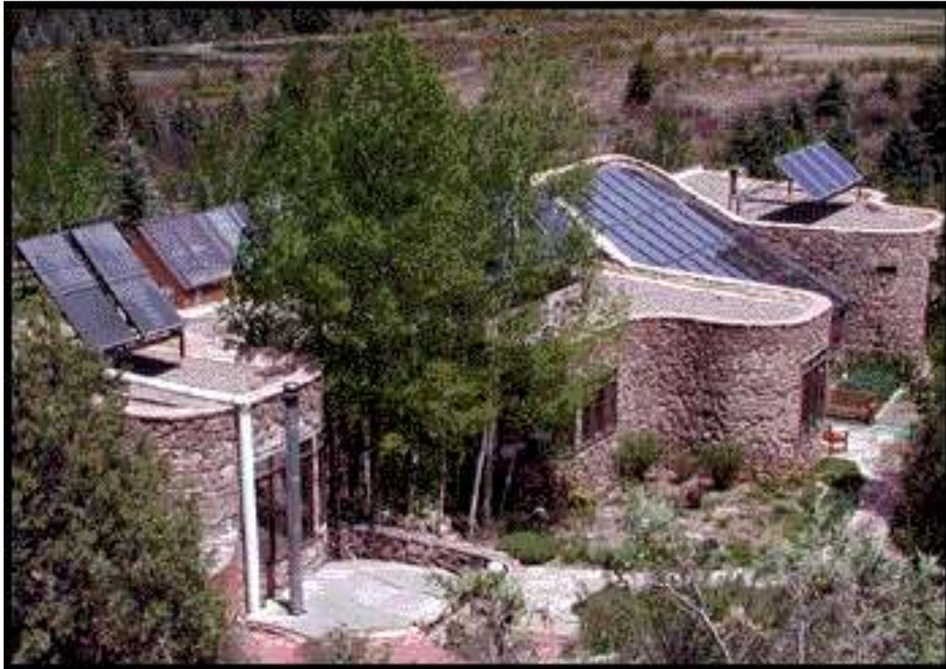
Single-storey 400 m<sup>2</sup> passive solar house and office building with superinsulated roof, walls, floor and windows. No backup space heating; small amount of LPG is used as backup to solar water heating and for cooking. Most energy usage is electricity for office equipment. “Zero net energy” since 1992.
